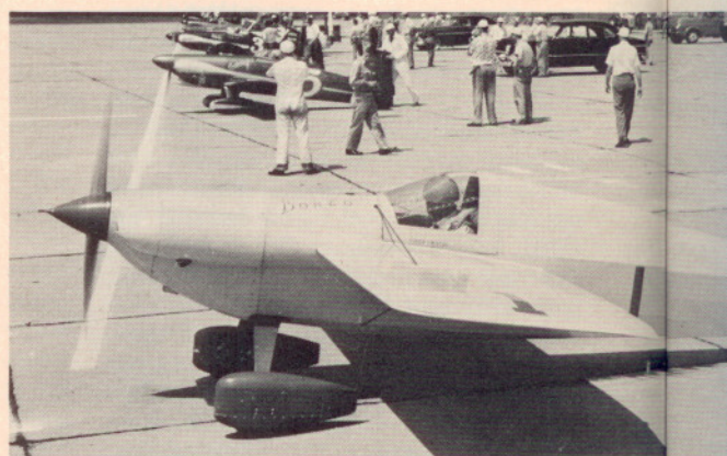
▲ First legalized homebuilts of the postwar years were the Goodyear racers introduced in 1947. The Wittman "Bonzo," shown in the photograph, is a sister ship of the 1947 winner, "Buster," itself converted from a higher-powered prewar design
