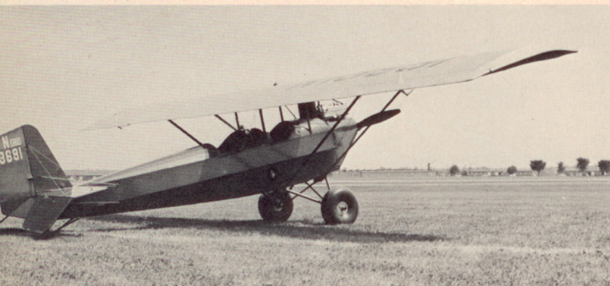
▲ The two-seat Pietenpol "Air Camper," powered with a converted Model A Ford automobile engine, was one of the most popular homebuilts of the 1930's. This one is a genuine antique but others are still being made from the 30-year-old plans
